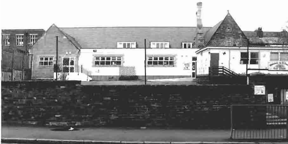
Fig. 14: St David's School, now disfigured by inappropriate modern alterations.
