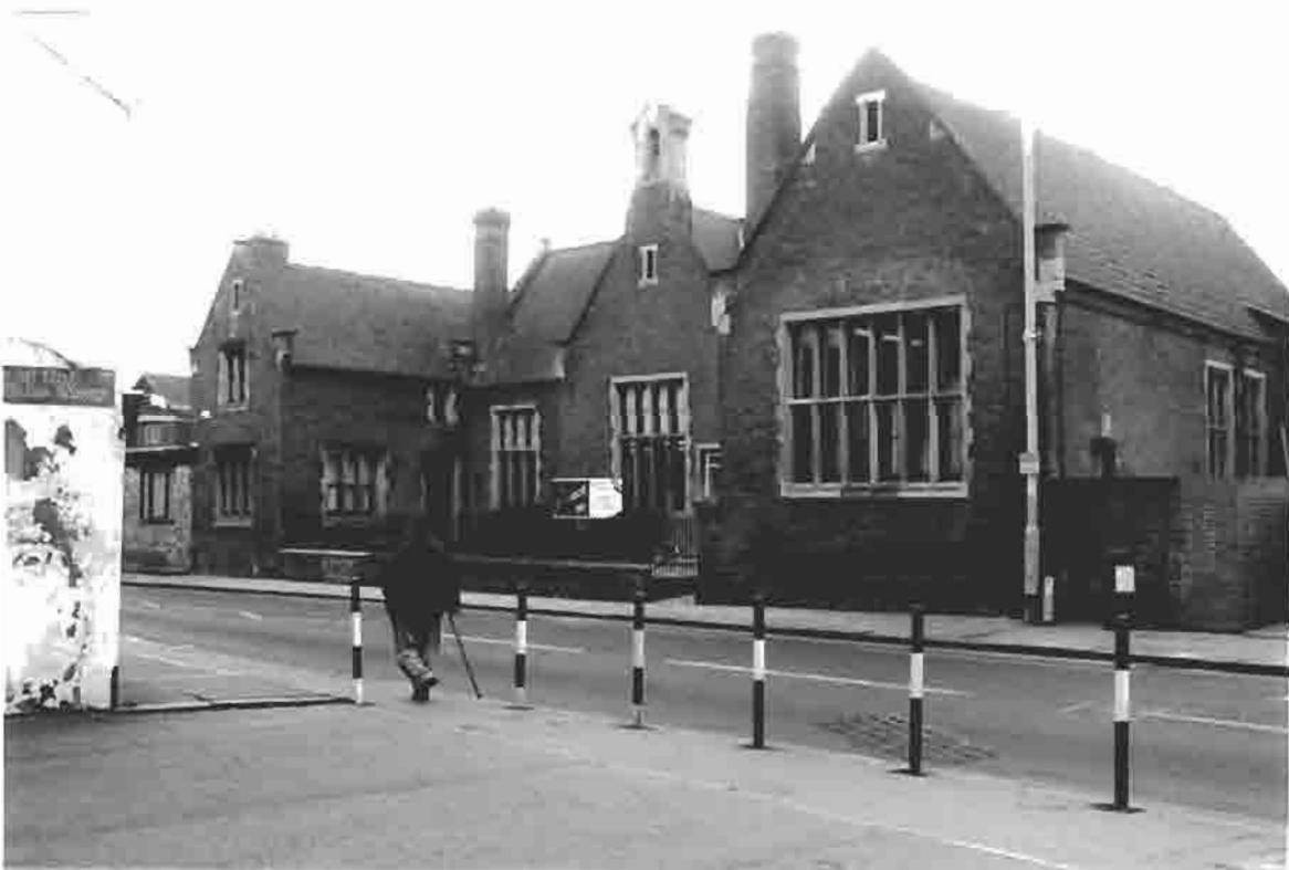
Fig. 12: Cowick Street First School, formerly St Thomas National Schools (A. Weslake 1861), showing the original school building on the left and centre, and the additional classroom of 1881 on the right.
