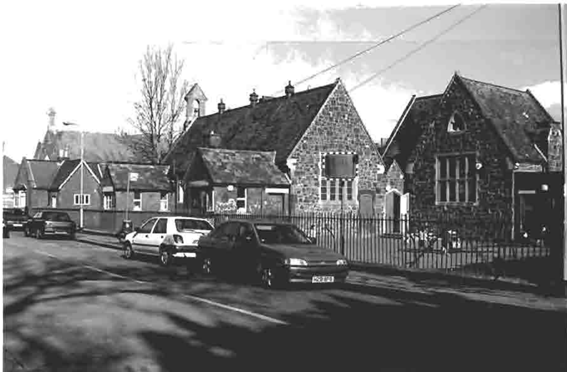
Fig. 9: The former Exwick National Schools (A. Weslake 1859-60), with the additional classroom of 1875 shown on the right.
