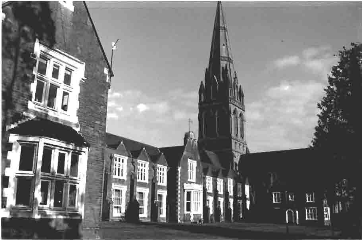
Fig. 10: The 1860s buildings of the former Episcopal Charity Schools (G.W. Cumming 1861-2), as altered in 1936-8 by the addition of an extra storey.
