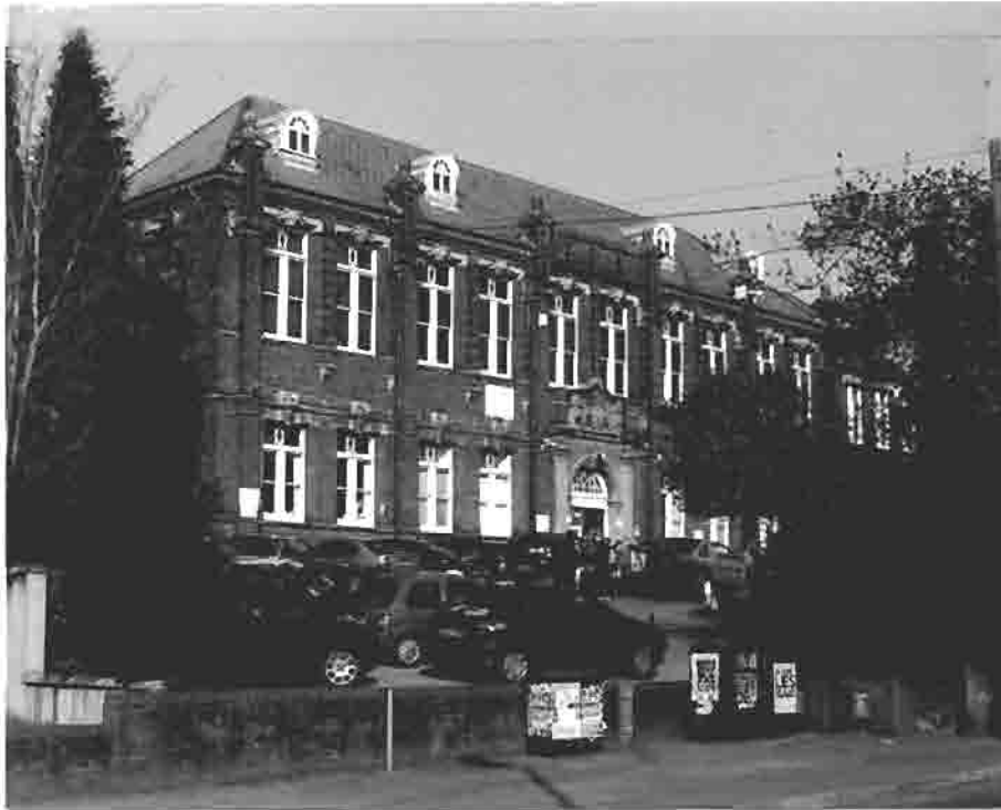
Fig. 23: The former Episcopal Middle Class School for Girls, now the Bishop Blackall Annexe of Exeter College (James Jerman 1884-8), restored after a fire in the 1980s, without its original central gable and cupola.
