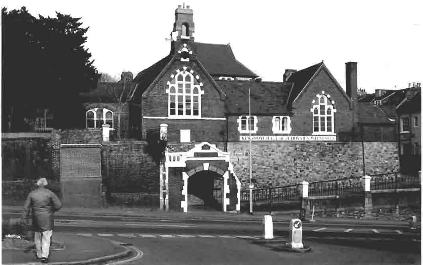
Fig. 18: The former Holloway Street Board Schools (Pearson Barry Hayward 1875-6), showing the original buildings of 1875 (with bellcote) at centre, and extensions of 1901 (with 'Kingdom Hall' signboard), at centre right.
