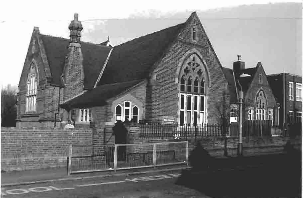
Fig. 16: The St Thomas Girls' Board Schools from School Road (R.M. Fulford 1872-3), showing the 1920s extension, on the site of the teachers' houses, at the extreme left. The infants' school, at the rear of the buildings, has been demolished.
