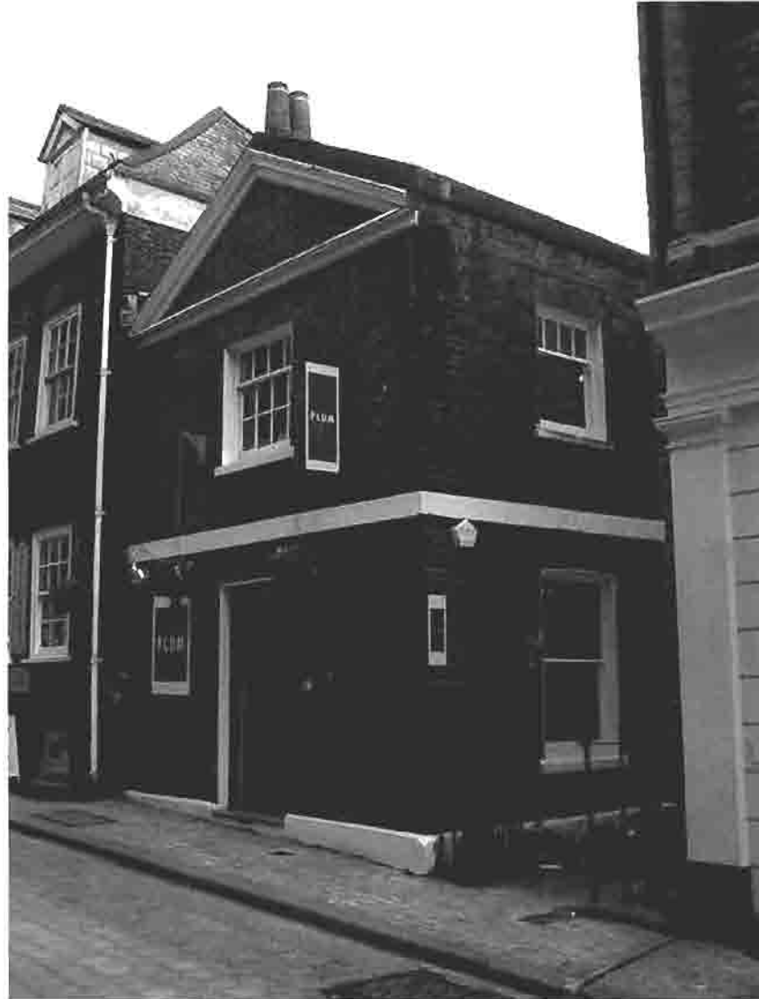
Fig. 1: Detail of one of the teachers' houses at the former Episcopal Charity Schools, Upper Paul Street
